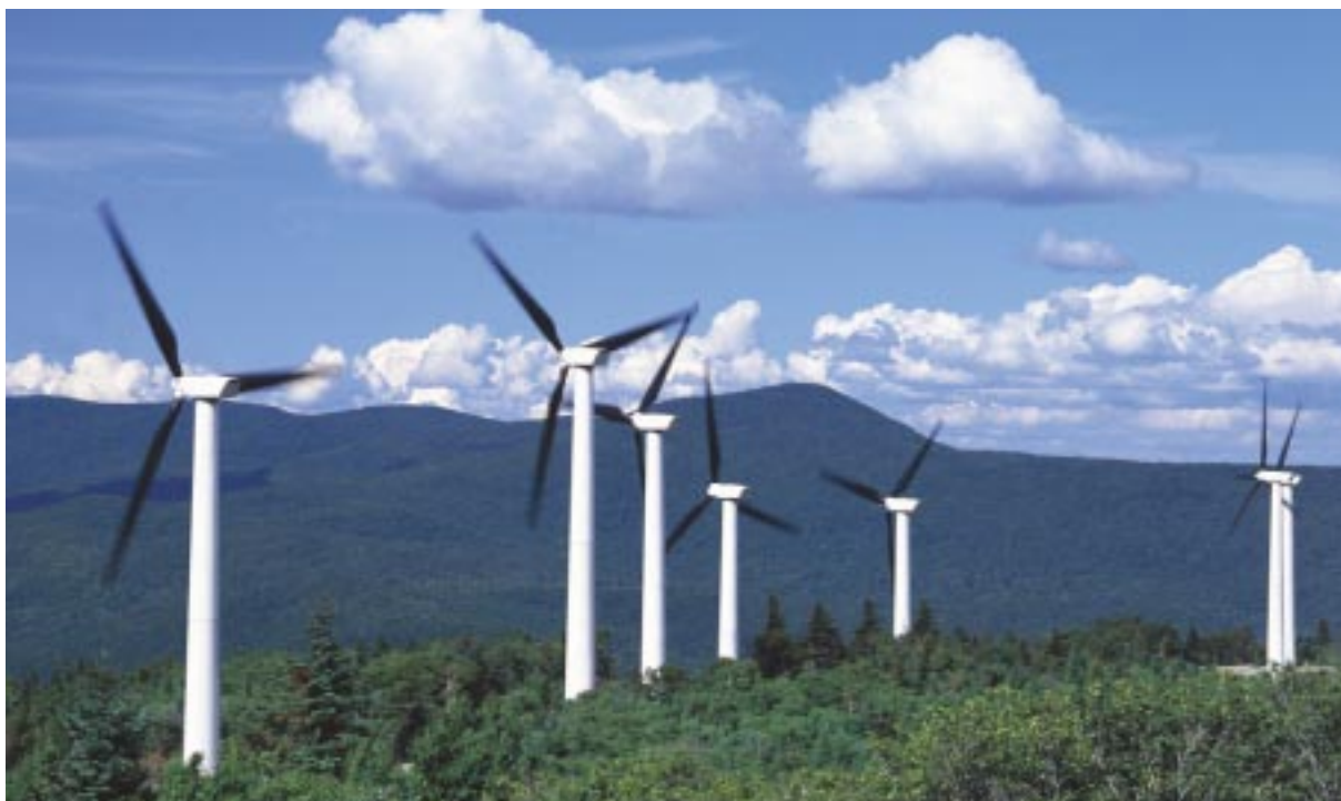
Photos: General Electric Company / Lloyd Herziger
